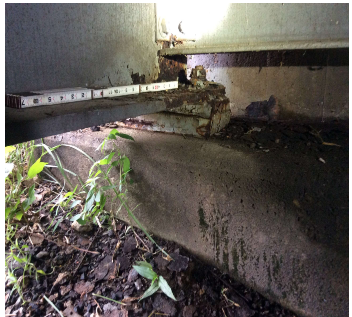
PHOTO 2 Description Span4 beam 1 pitting to web and bottom flange up to 3/16".
