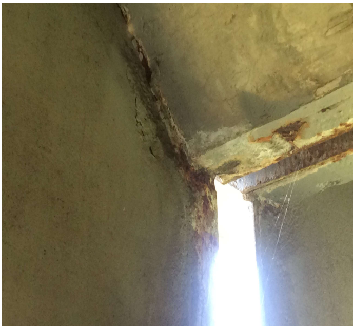
PHOTO 1 Description Painted over section loss on beams with minor rust
