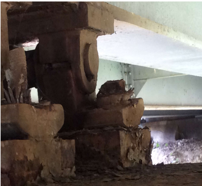
PHOTO 1 Description Span 1 bearings under girders 1,2,4 and 5 has up to 3/8 inch gap around bearing pin
